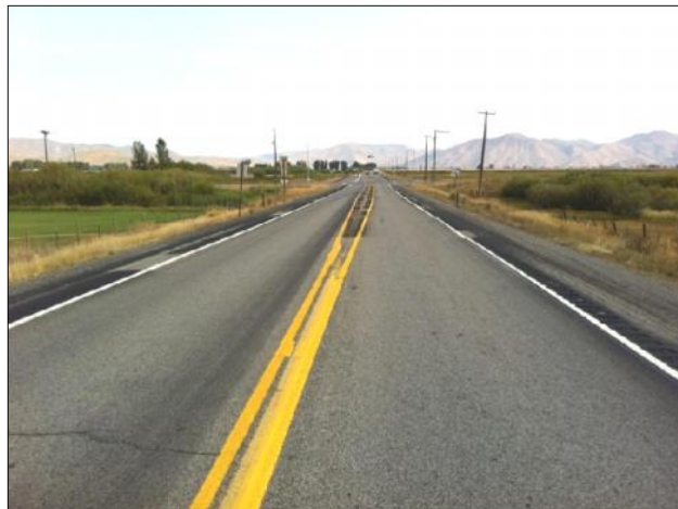
Figure 1. Lane narrowing on SH-75.
