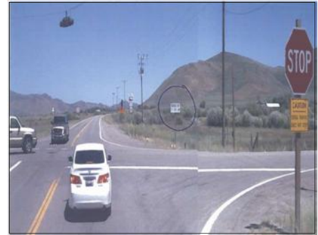
Figure 3. Example of sign clutter EB on US-20. Buckle up sign has been removed. Cross Traffic Does Not Stop Sign has been enlarged.
