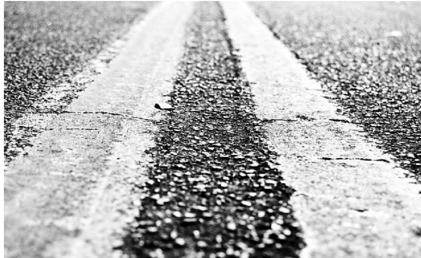
Paint sticks best to pavement that is neither too rough nor too smooth.
