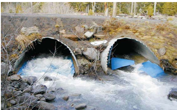
Culverts protect roadways by channeling and slowing water flow, thus reducing erosion.
