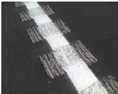
A four-inch edge line rumble stripe placed on a rural highway in Iowa
