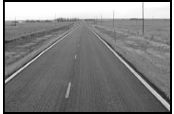
Typical rural highway where the last pavement overlay left no shoulder area.
