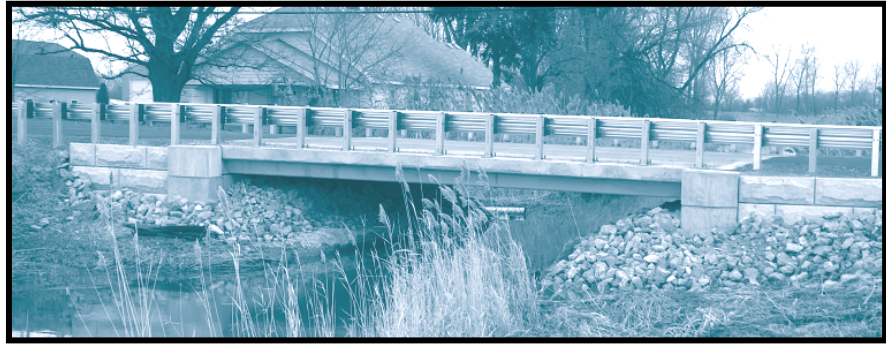
The new Suder Ave. Bridge in Monroe County
