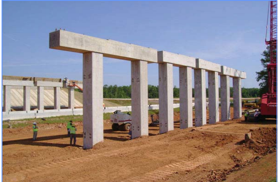
Example of accelerated bridge technology
