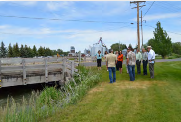
Eagle Rock Bridge , Bonneville County
