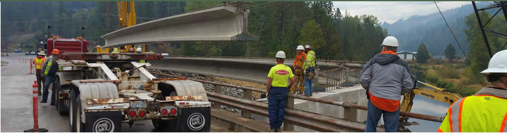
Enaville Bridge, Shoshone County Road and Bridge
