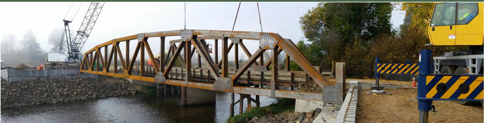
Middle Fork Payette River Bridge, Boise County
