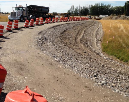
Slope improvement Bingham County
