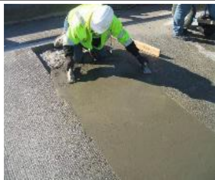
Concrete Deck Patching
